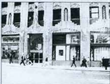
Elegant entrance: where the energy is...
